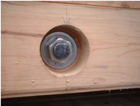
Beams are bolted together with countersunk nuts.
