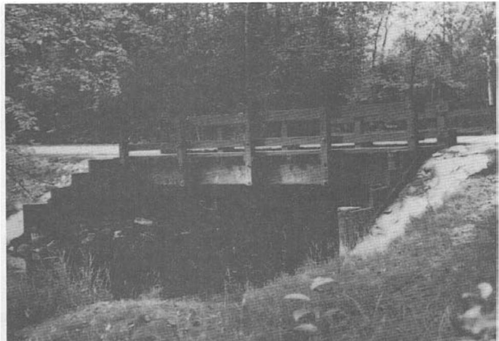
*Figure 2-5.- Typical sawn lumber beam bridge. Most lumber beam bridges of this type span 25 feet or less, but longer spans have been built where large beams are available.*
