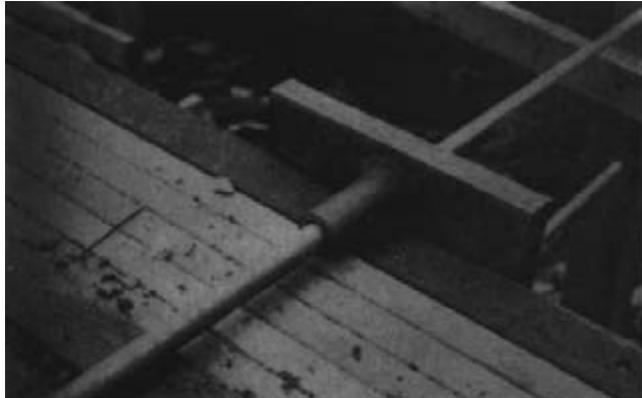
*Figure 15-40. - Prestressing anchorage used at the Pickerel River Bridge.*
