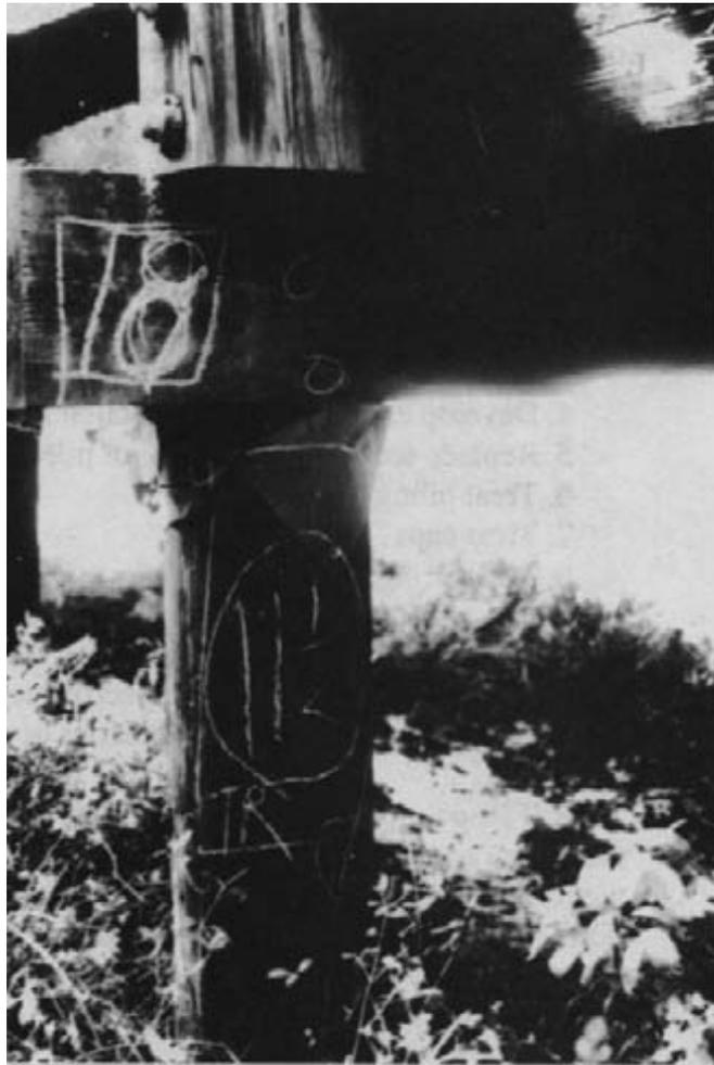
*Figure 15-1. - Typical investigative borehole pattern.*
