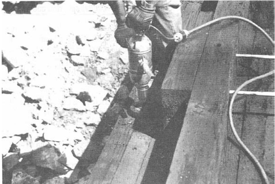
*Figure 5-31. - Field-grooving for a split ring connector for a curb-deck attachment. Field fabrication such as this requires field treating with wood preservative, as discussed in Chapter 12 (photo courtesy of Wheeler Consolidated, Inc.).*
