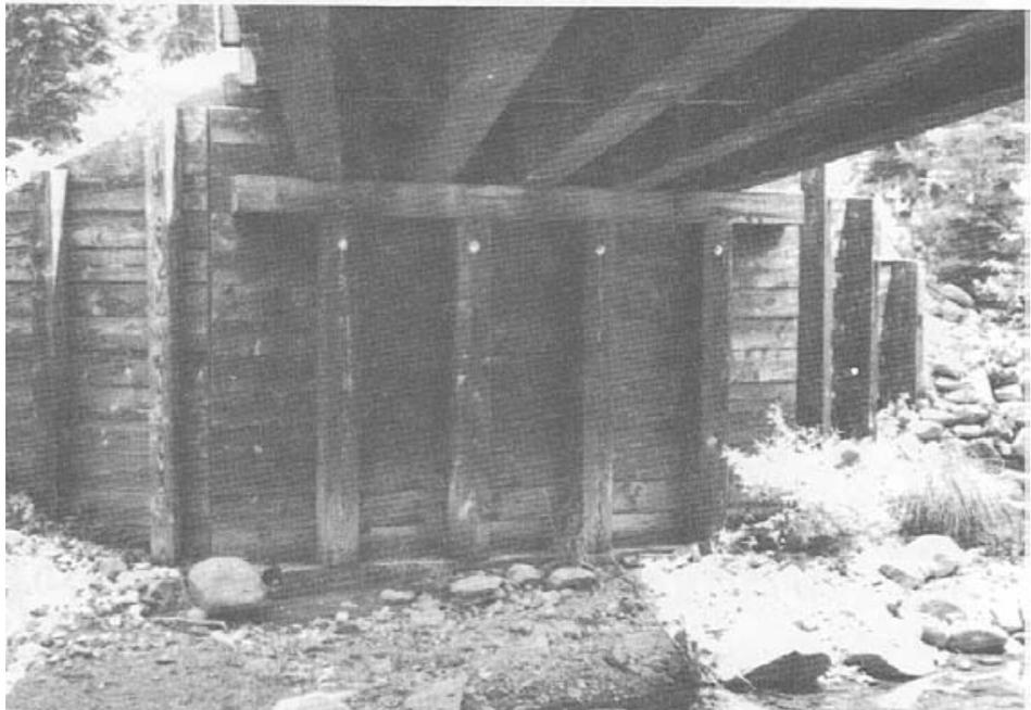
*Figure 2-31.- Sawn lumber post abutment.*
