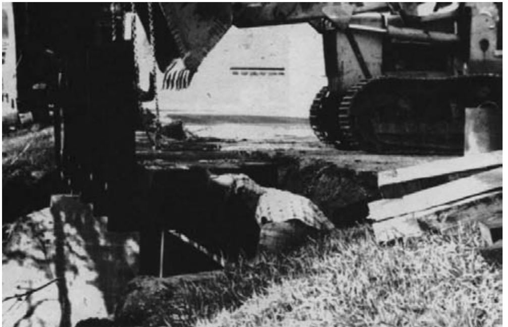
*Figure 15-23. - A prefabricated deck panel is lifted onto the abutments. Each panel was prefabricated to fit each bridge.*
