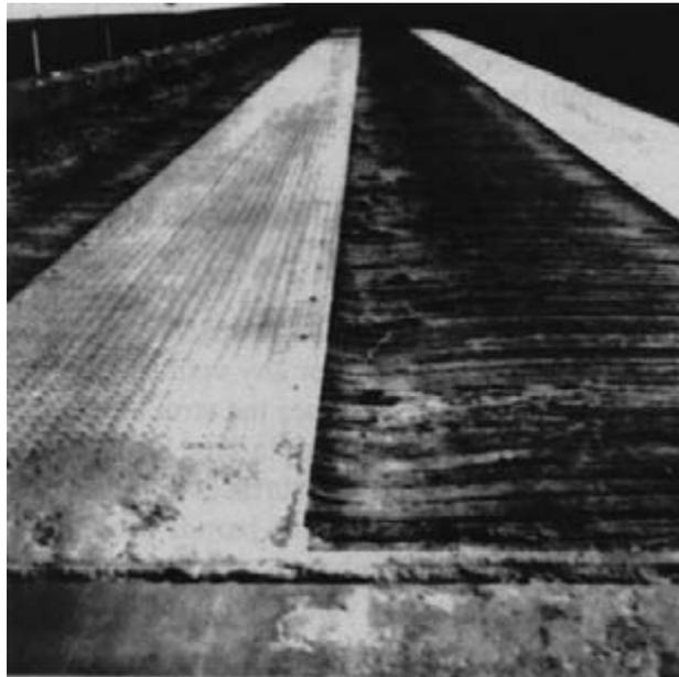
*Figure 11-2. - Severe abrasion on a nail-laminated lumber deck caused by vehicles off-tracking the partial steel plate wearing surface (photo courtesy of Sakee Poulakidas, USDA Forest Service).*
