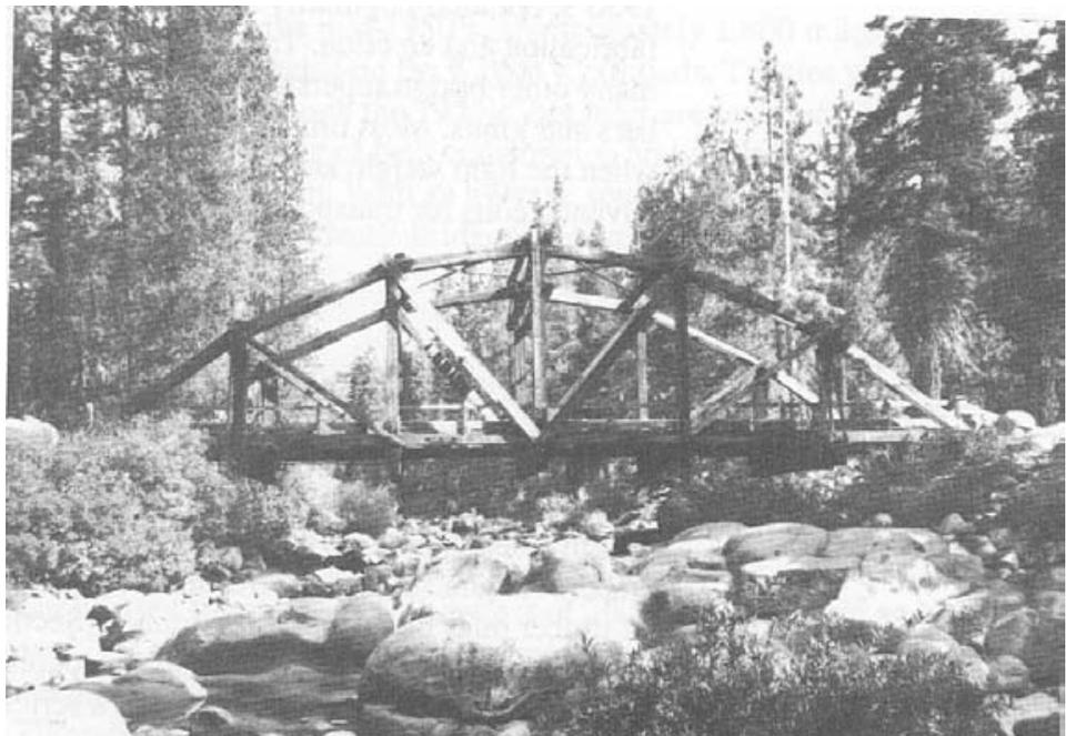
Figure 2-14.- Lumber bowstring truss over Dinkey Creek on the Sierra National Forest in Central California. This truss spans 90 feet and was built in 1934 (photo courtesy of Raul Gonzalez, USDA Forest Service).
