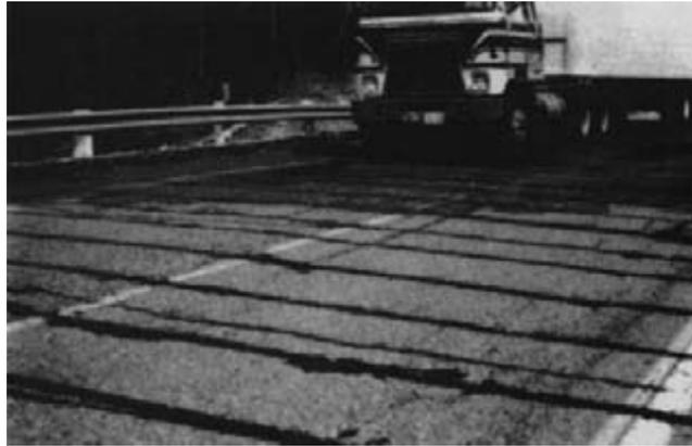
*Figure 15-42. - Top prestressing bars installed in grooves cut in the asphalt wearing surface of the North Pagwachuan River Bridge near Terrace Bay, Ontario.*
