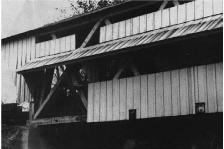
*Figure 15-34. - Completed repair of one corner of the bridge, using poplar timbers. Note the closer spacing of the endmost floorbeams to account for the reduced floorbeam load distribution adjacent to the abutment.*
