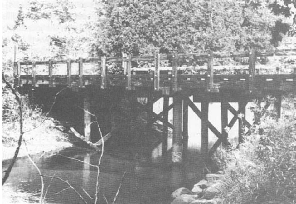
*Figure 2-10.- Longitudinal glulam deck bridge over Au Train Creek on the Hiawatha National Forest. This bridge is 58 feet long over three spans and supports a 26-foot roadway width.*
