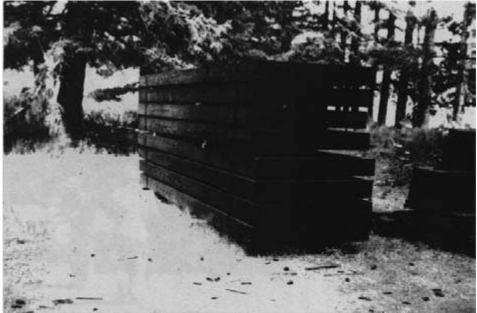
*Figure 12-9. - Glulam deck panels stacked for storage.*
