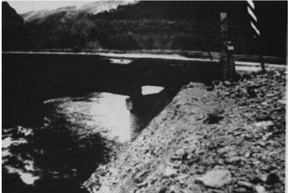
*Figure 15-58. - The temporary repair made to the bridge consisted of replacing the approach embankment and lifting the nail-laminated approach span back into position.*
