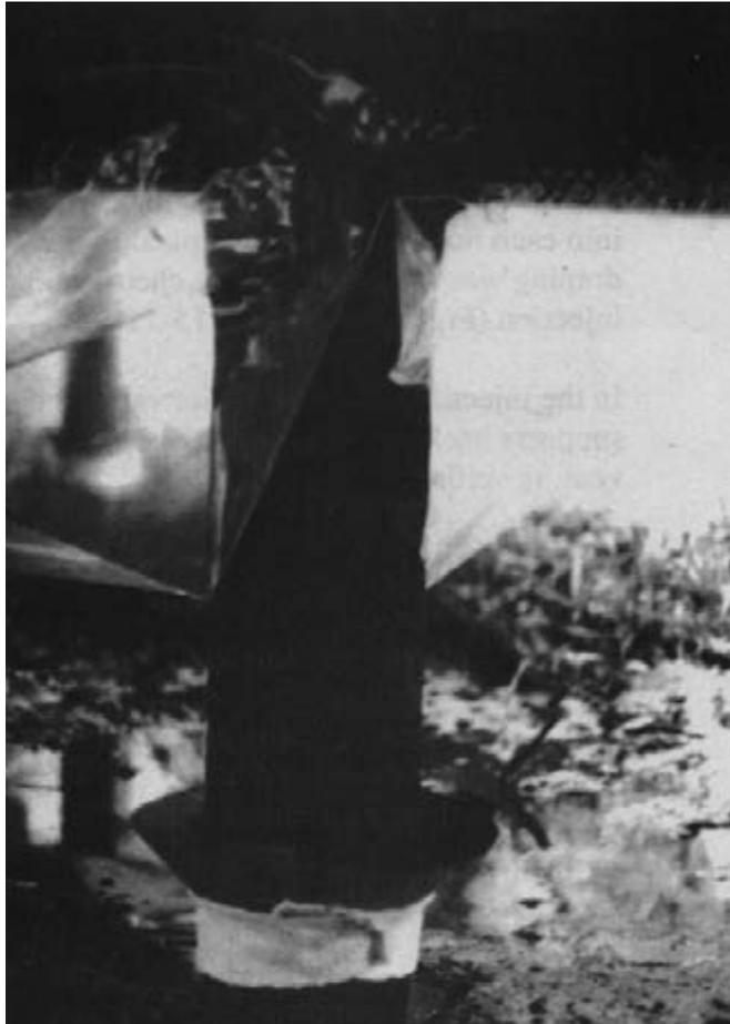
*Figure 15-10. - Typical individual cap and pile draping and funnel for protection against leakage of the liquid preservative.*
