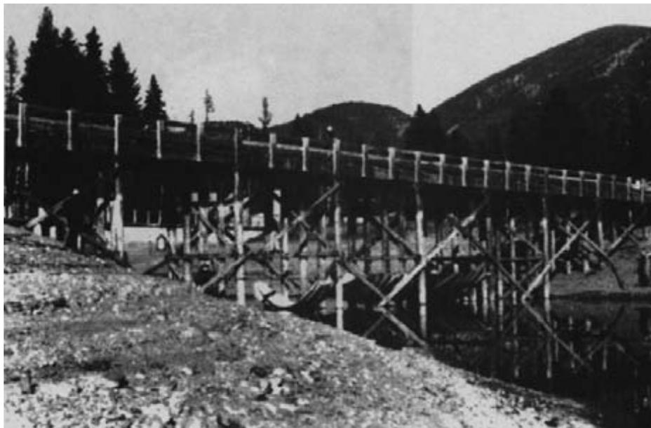
*Figure 15-13. - View of the Sullivan Lake Outlet Bridge as in-place treatment was commencing. Note the canvas slings placed under the bridge to prevent water contamination should accidental spillage of treatment chemicals occur.*
