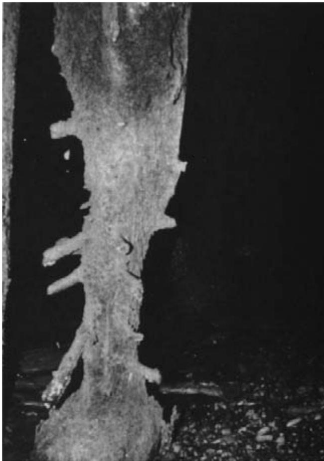
*Figure 13-18. - Limnoria damage to a timber pile, evidenced by the characteristic hour-glass shape in the tidalzone.*
