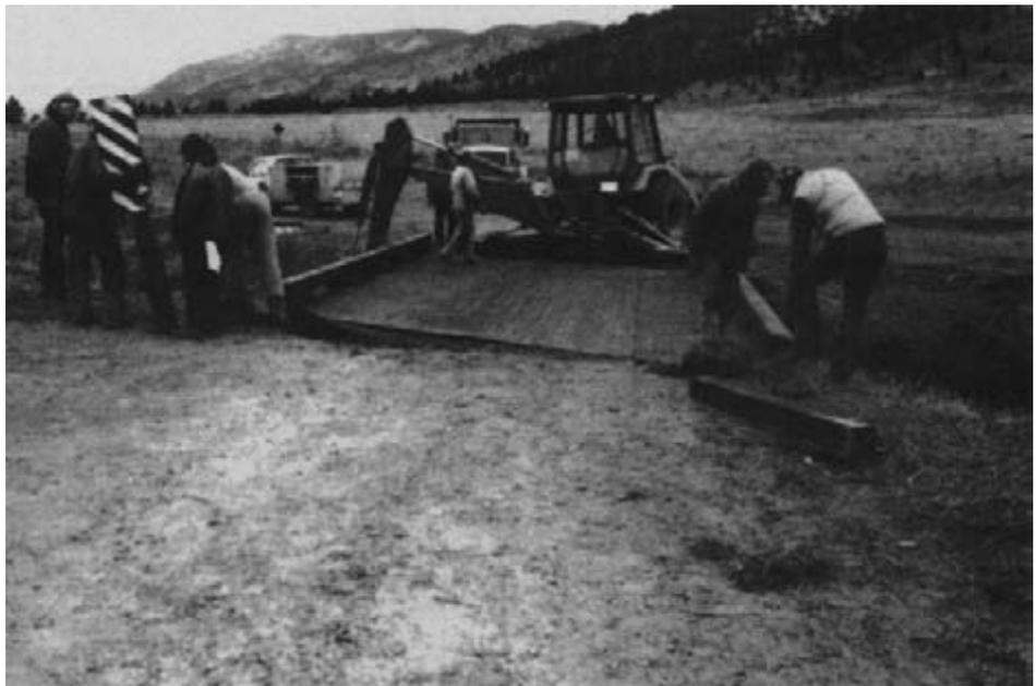
*Figure 15-74. - Curbs are attached to the deck.*
