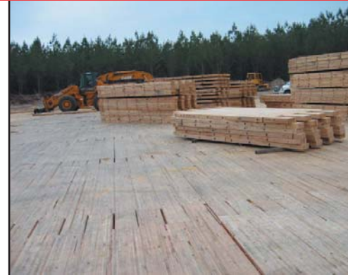
Drill site being prepped with emtek mats.
