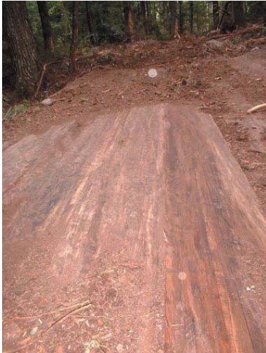
Mat surface after 18 months of continuous use under skidder chains.
