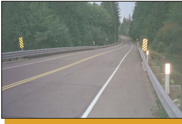
Figure 10—Crack-free deck on the Lighthouse Bridge near Port Angeles, WA.
