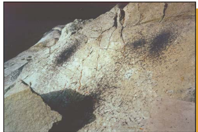
Figure 24b—Asphalt dripping onto rocks under the Shady Cove Bridge.
