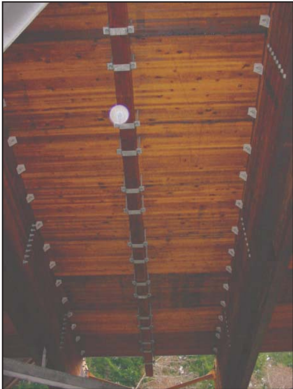
Figure 5—Distribution beam installed under the Satsop River Bridge.
