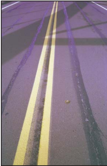
Figure 4—Longitudinal cracks over the deck panel joint on the Satsop River Bridge near Shelton, WA.
