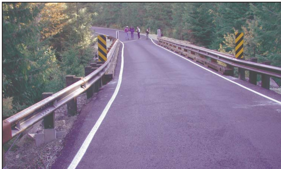
Figure 1—Paved timber bridge in Oregon.
